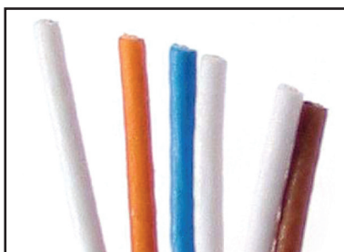
9. Trim ends of orange, blue and brown pairs at slight angle to make loading easier
